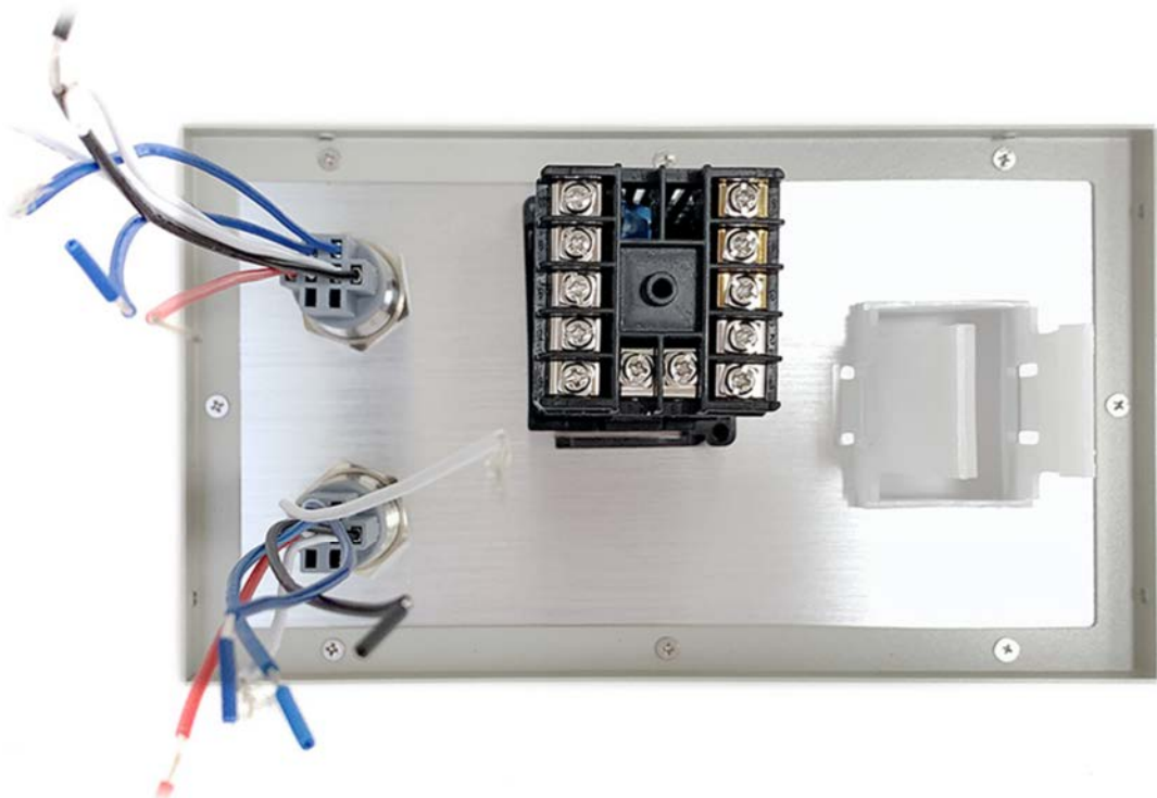
Figure 20. Add wiring harness to the switches and mount breaker bracket.
